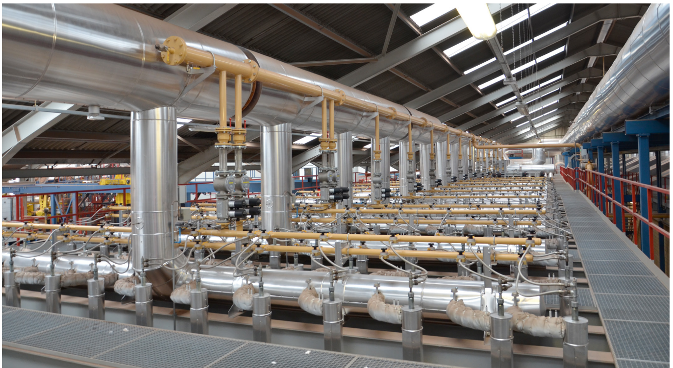
Top of Tunnel Kiln
