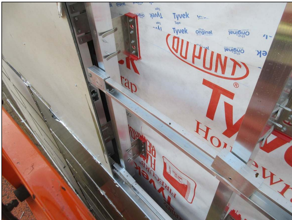
TEST SAMPLE DURING DISMANTLE
