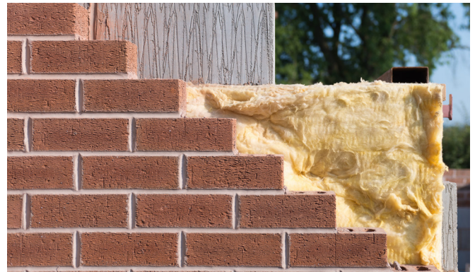
Full fill mineral wool insulation
