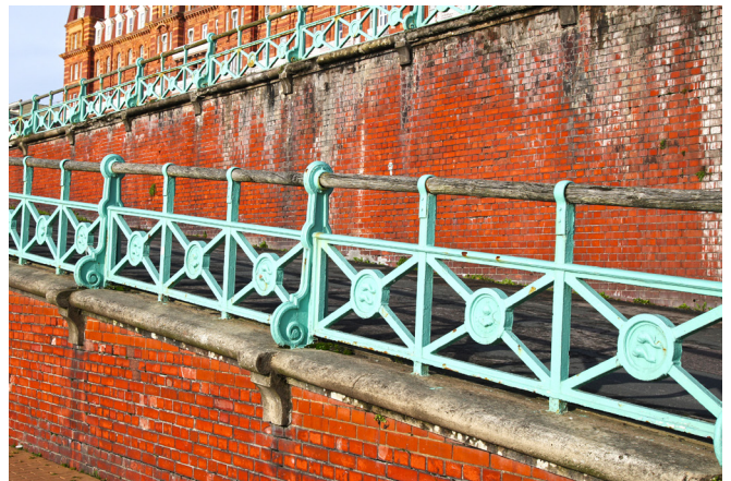
Brickwork exposed to a marine environment
