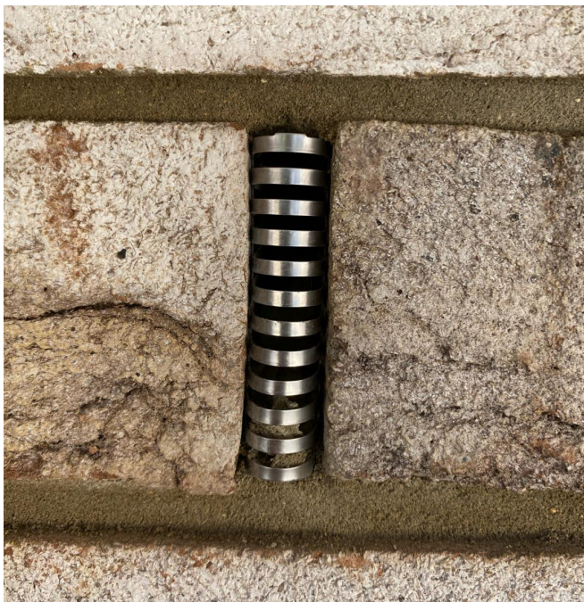
Stainless steel weep vent
