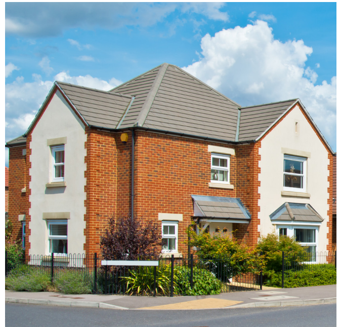
Render and brickwork cladding
