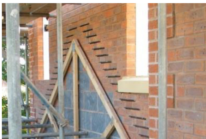
Stepped cavity tray for pitched roof
