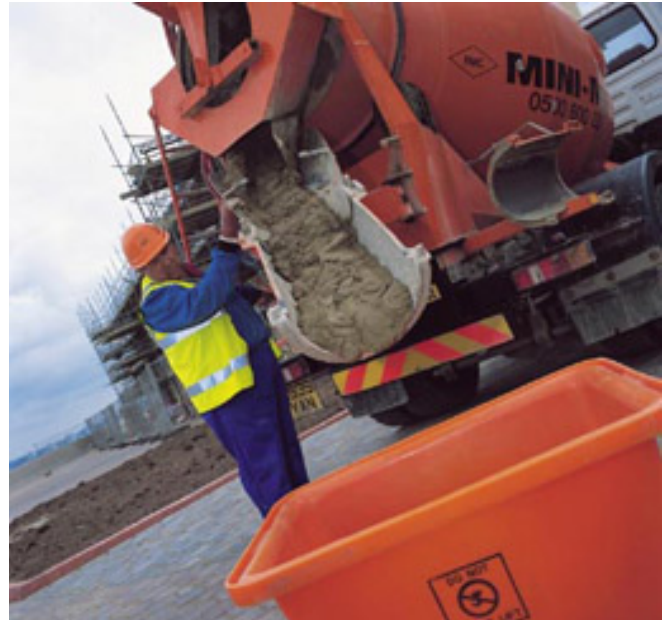
Mortar being delivered to site
