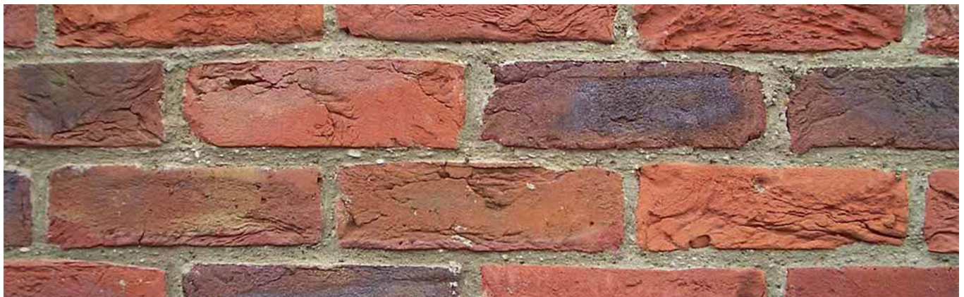
Mortar choice can have a big visual impact on brickwork
