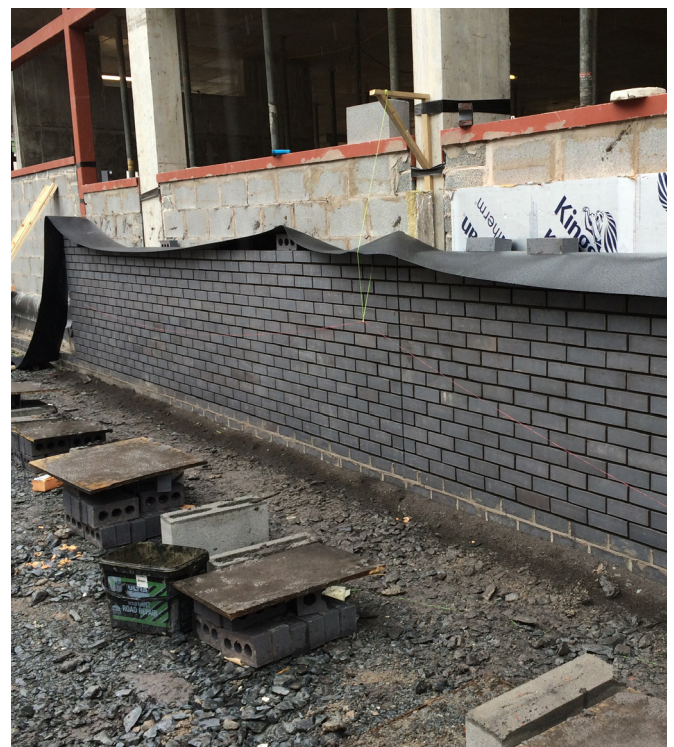
Protecting mortar from inclement weather is essential
