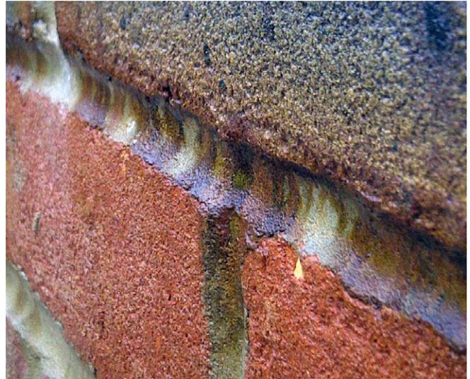
Iron staining visible on a mortar joint
