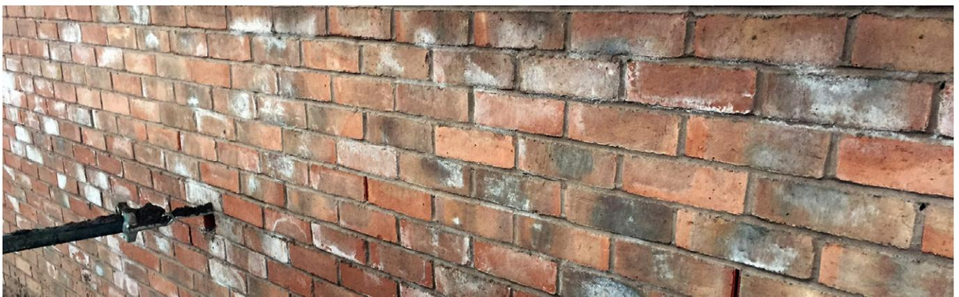
Efflorescence on brickwork under construction
