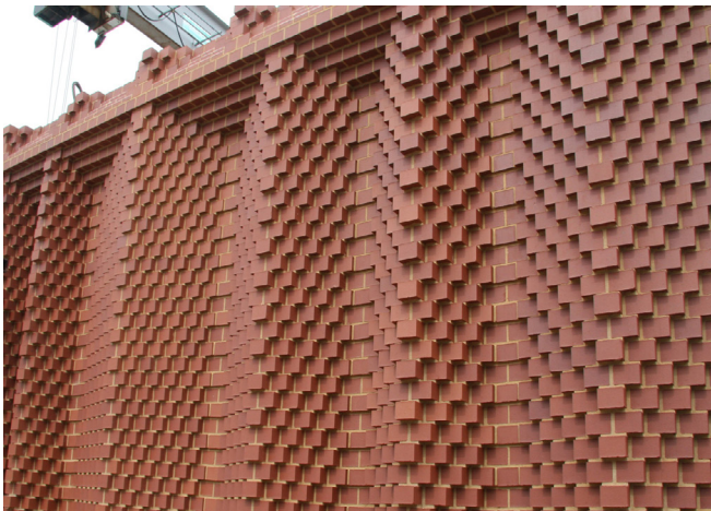
Precast panels with engineering bricks
