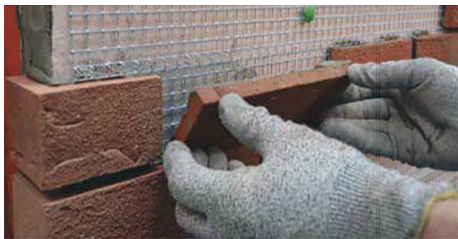
Mesh backing board to improve adhesion
