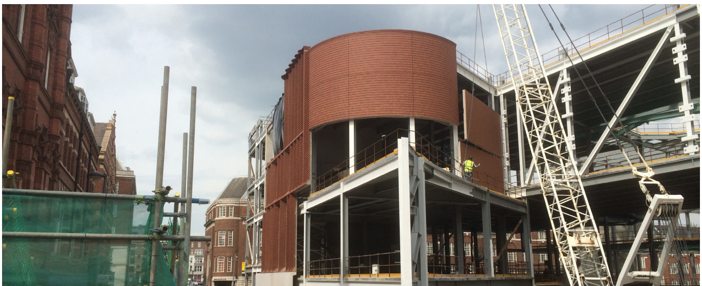
Panels can be fixed to a variety of frame types
