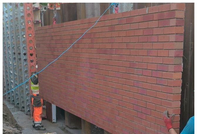
Single skin prefabricated brickwork
