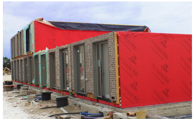
Panel system on 3D primary structure
