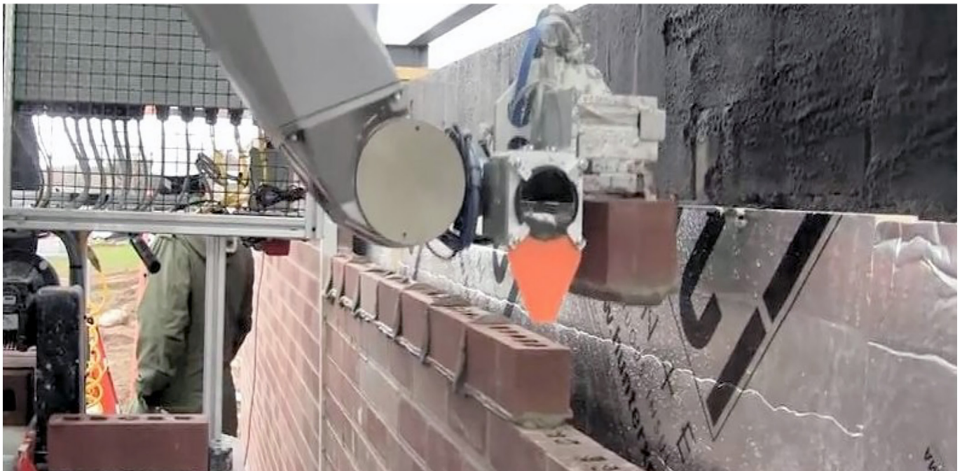
Sam 100 Bricklaying robot in action
