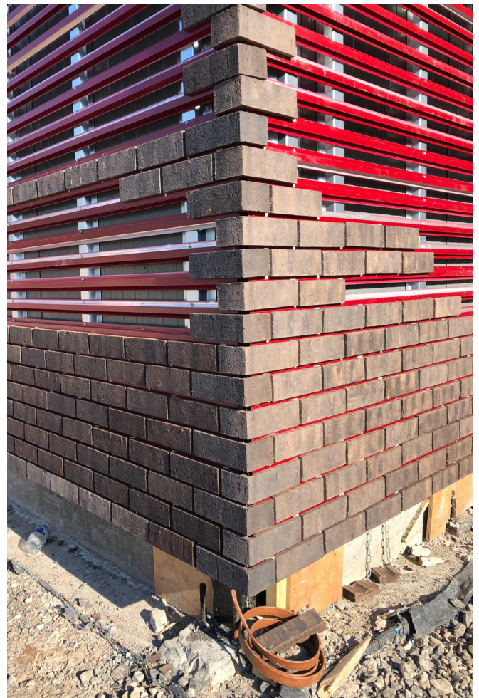
Rail system to achieve mechanical fixing
