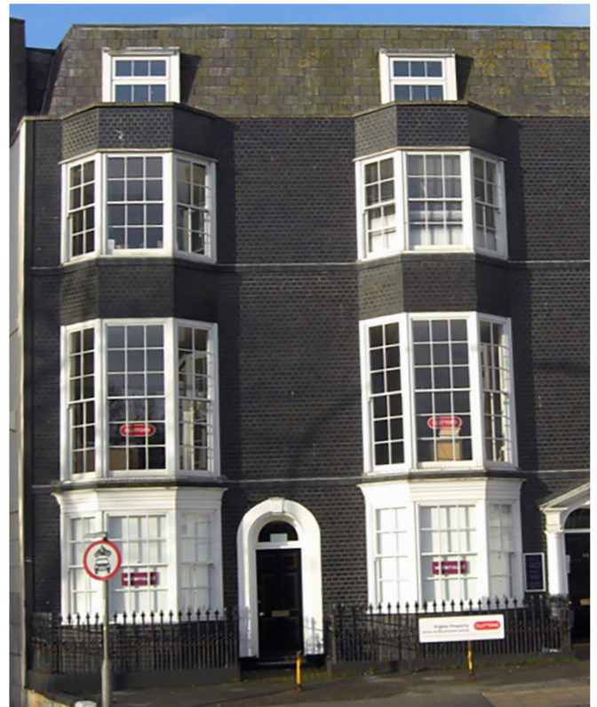
Timber framed property clad in mathematical tiles
