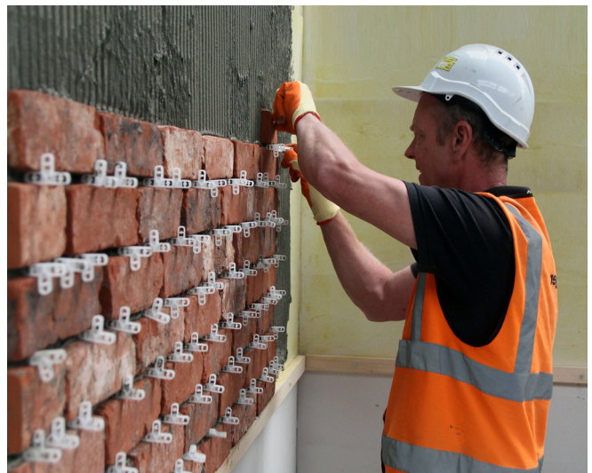
Brick slips used internally
