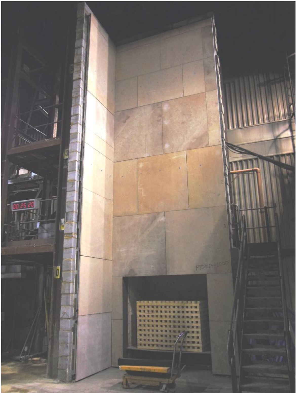
Figure 2. Full-height photograph of cladding system prior to test.
